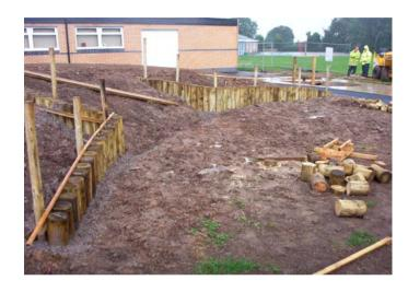
An existing topsoil/subsoil mound was reduced in size and re-graded. The facilities constructed included a rock/pebble water feature using river washed cobbles set into a concrete base which formed a pool area and stream. This stream was bridged with a timber boardwalk. The water feature was fed via a connection to the building water mains.
