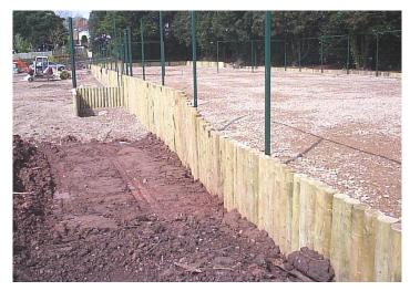
Tree clearance works were followed by the excavation of the three existing courts and a reduction in subsoil levels to form two tiers.
